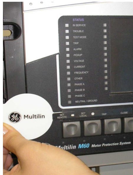
Figure 4-21: STEP 3 - PULL THE TOOL OUT WITH THE PUSHBUTTON LABEL
