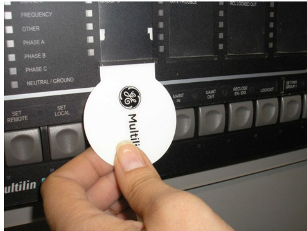
Figure 4-14: STEP 2 - SLIDE THE TOOL IN UNTIL THE TABS SNAP OUT AS SHOWN
