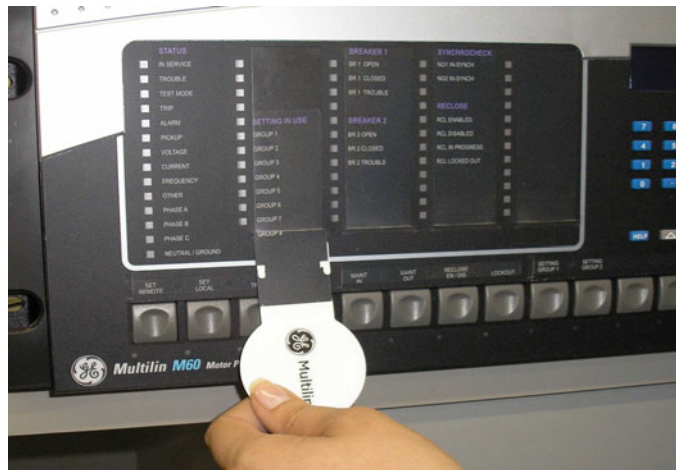
Figure 4-15: STEP 3 - PULL THE TOOL OUT ALONG WITH THE LED LABEL
