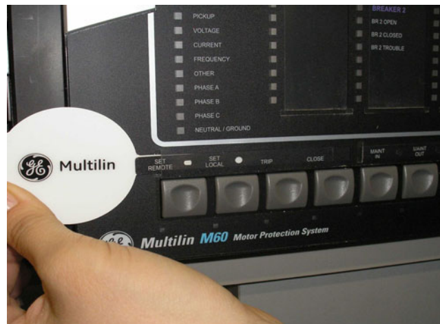
Figure 4-20: STEP 2 - SLIDE THE TOOL IN UNTIL THE TAB SNAPS OUT AS SHOWN
