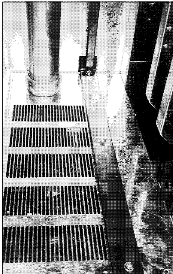
Fig. 32 Main Ground Bus
