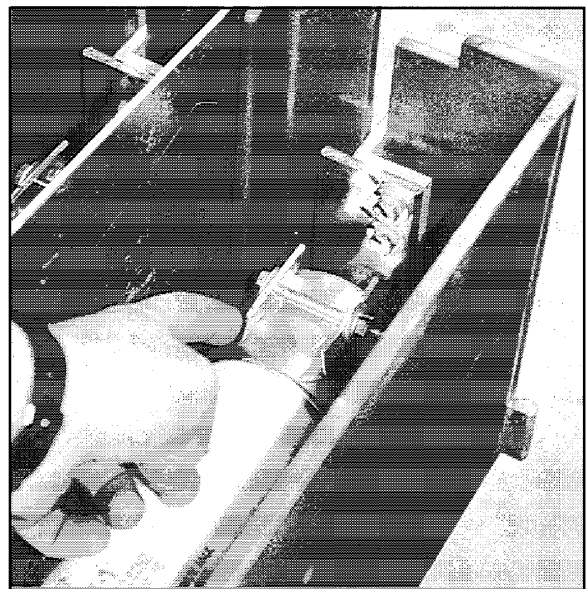
Fig. 61 Examine Fuse Clips
