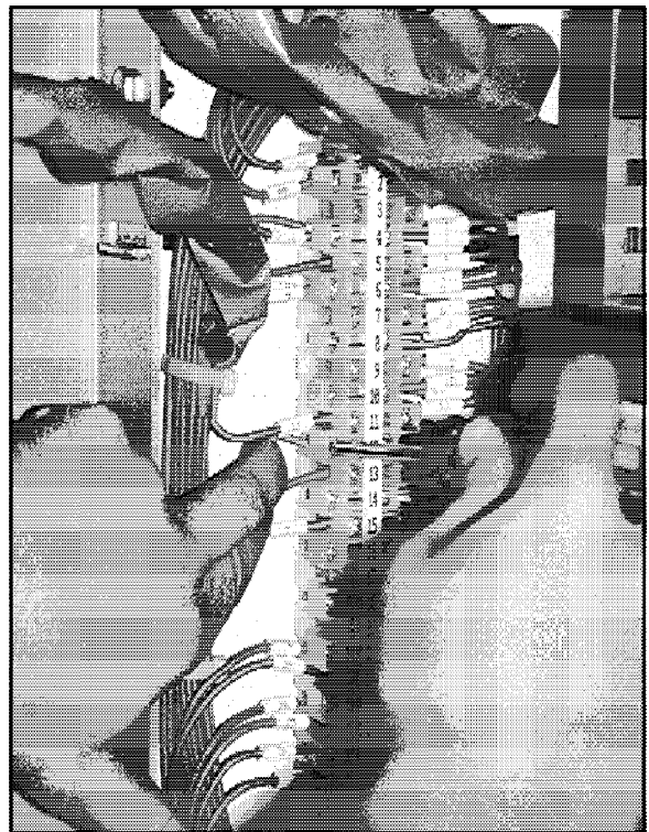
Fig. 42 Removing Current Transformer Shorting Jumpers
