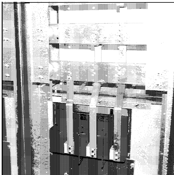
Fig. 55 Check Electrical Joints
