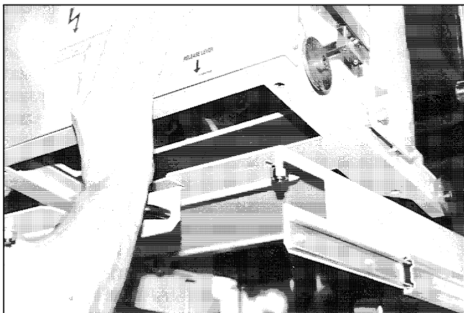
Fig. 47 Placing The Contactor On The Service Drawer
