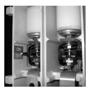
Figure 10 - Open contactor - OFF indication
