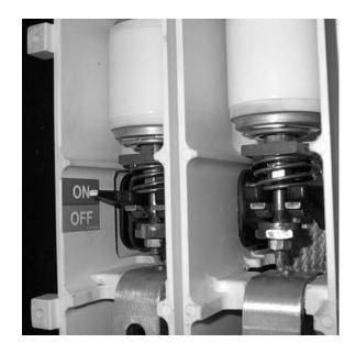
Figure 9 - Closed contactor - ON indication
