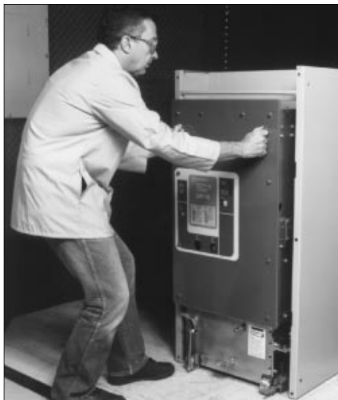
Figure 4-9 Positioning of 5 kV DHP-VR Breaker
