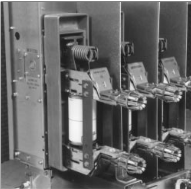
Figure 5-1 DHP-VR 5k V Interrupter Assembly
