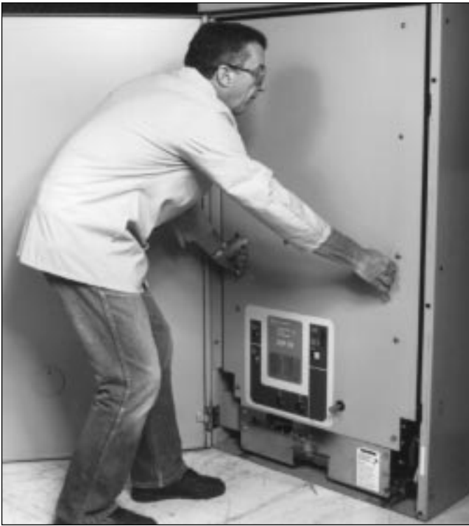
Figure 4-10 Positioning of 7.5 or 15 kV DHP-VR Breaker
