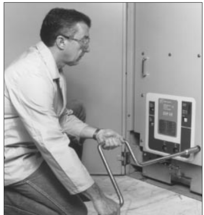
Figure 4-14 Levering 7.5 or 15 kV Breaker to Connected Position
