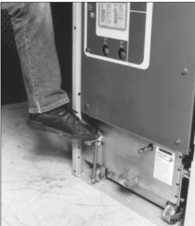
Figure 4-11 Final Engagement of 5 kV Secondary Contact
