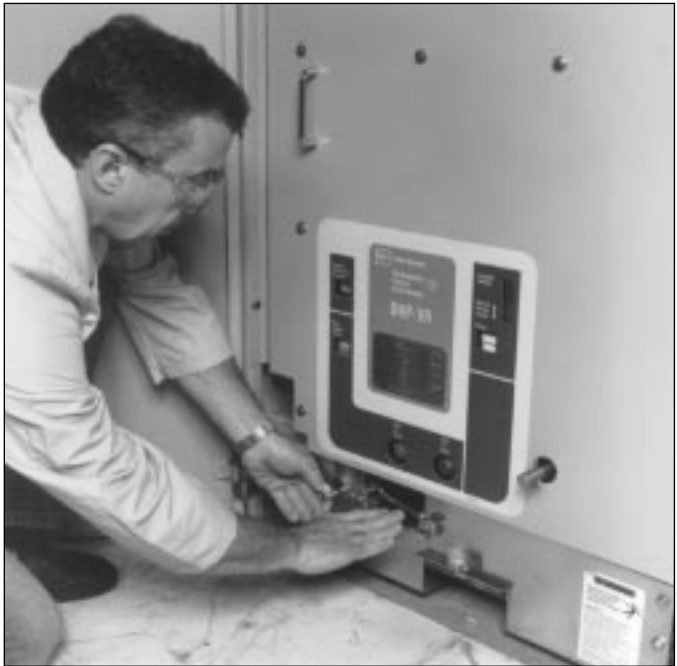
Figure 4-12 Final Engagement of 7.5 or 15 kV Secondary Contact
