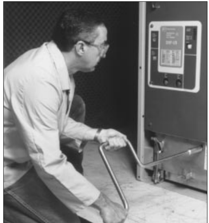
Figure 4-13 Levering 5 kV Breaker to Connected Position
