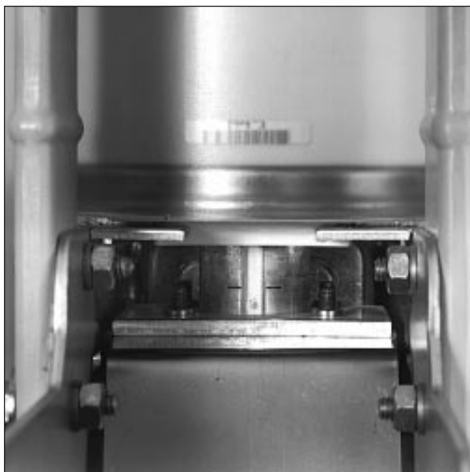
Figure 7-2 Vacuum Interrupter Showing Contact Erosion Indicator with Breaker Open (Shown Here for Clarity Purposes Only)
