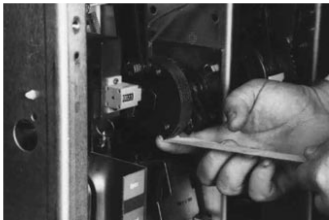
Figure 6-6 Starting Tape at Bottom of Cam
