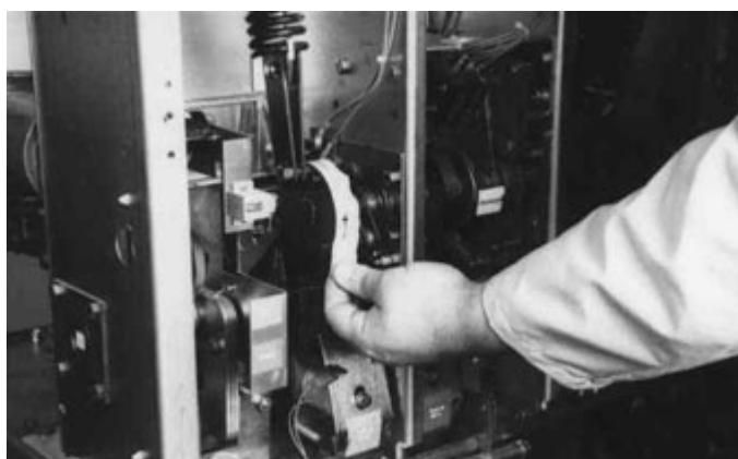
Figure 6-16 Remove Marked Masking Tape from Cam
