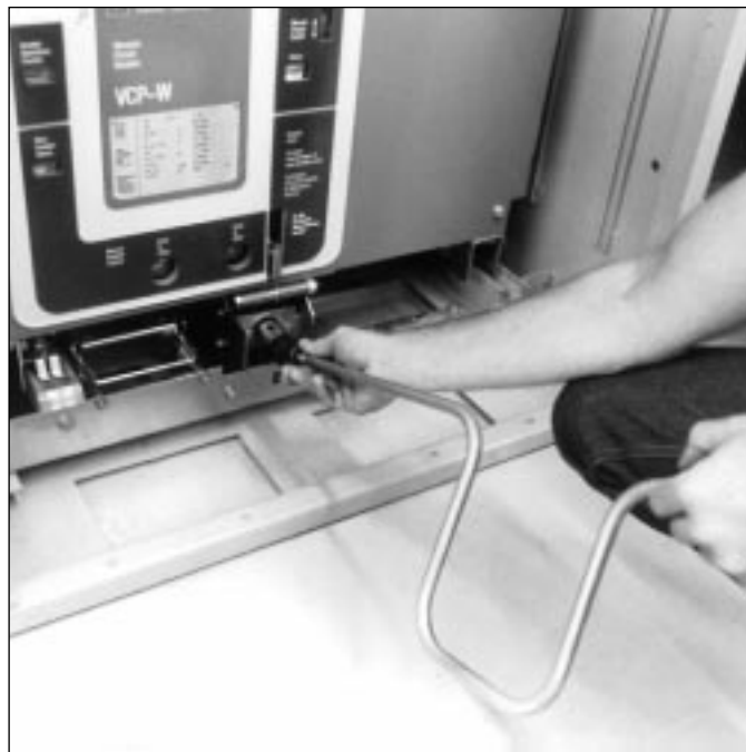
Figure 4-6 Engaging Levering-In Crank
