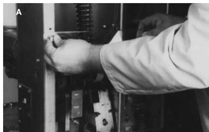
Figure 6-9 Attaching CloSure™ Test Tool at Hole “A”
