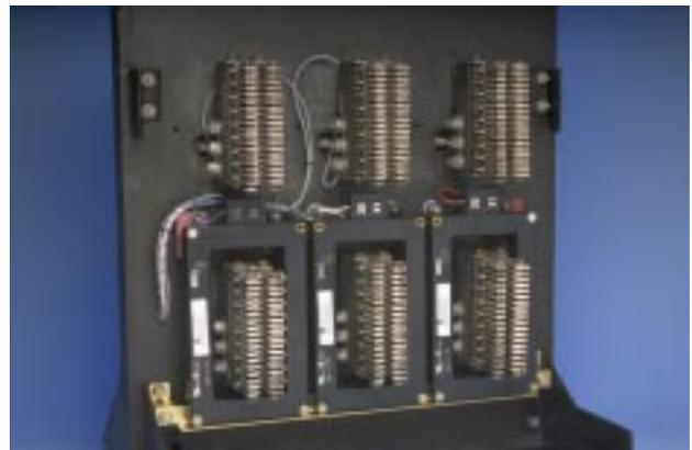
H. Turn the two (2) nylon screws, located in the upper corners of the Sensor Assembly, until they have started in the threaded holes in the Glass Poly Sensor Mounting Plates. Continue turning the screws until the Sensor Assembly is parallel to the Breaker Back Plate. Do not over-tighten the screws. Once the Sensor Assembly is parallel to the Breaker Back Plate, tighten the nuts previously installed on the nylon screws against the Sensors to lock the screws in place.
