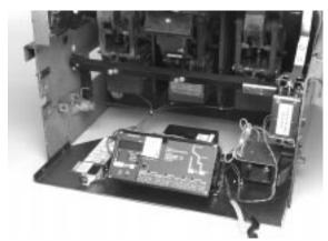
NOTE: For Steps 13 A through C, position the Trip Unit Mounting Platform Assembly in front of and as close to the Breaker as possible while still providing access to the components inside the Breaker.
