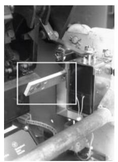
NOTE: The Trip Finger Assembly is supplied with the Shunt Trip Bracket installed. If the Breaker being Retrofitted was not equipped with the optional Shunt Trip, remove the Shunt Trip Bracket before installing the Trip Finger Assembly.
