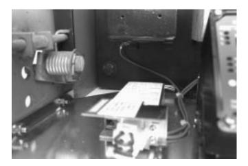
D. For Kits Supplied with a Breaker Mounted CPT Only: Route the Line Side HV Wires along the same path as the Sensor Harness.
