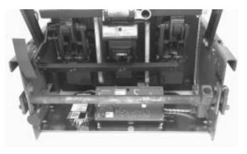
F. Route the External Harness towards the right side of the Breaker, then up towards the DTA Assembly. Remove the top front screw securing the DTA Mounting Bracket. Using the two wire clamps and the screws supplied, secure the External Harness to the DTA.
