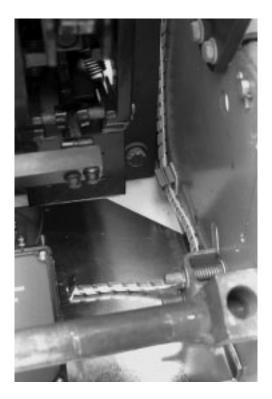
B. Route the DTA Wires downward to the Aux. CT Module. Connect the DTA Wire marked "+" to the "OP" and the unmarked wire to the "ON" terminals of the Aux. CT Module.
