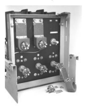
Attach the appropriate label for the Breaker to the Breaker in a clearly visible position. Three (3) labels are included with the CPT, one (1) for 480 Volt, one (1) for 240 Volt, and one (1) for 208 Volt systems.
