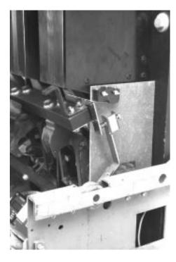
A. Align the holes in the Glass Poly Barrier Mounting Bracket with the holes drilled in the right Breaker Frame in Step 8. Mount the Glass Poly Barrier to the Breaker Frame, as shown, using the (2) .190-32 x .500" screws, (4) flat washers, (2) lock washers, and (2) nuts supplied.
