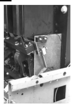
H. For Kits Supplied with a Breaker Mounted CPT Only: Route the Line Side HV Wires along the right rear side of the Breaker to the bolts below the top Breaker Stabs.
