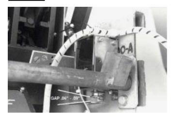
Step 13: Installing the Trip Unit Mounting
