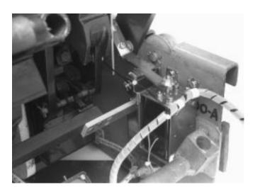
G. For Kits Supplied With An Auxiliary Switch Only: Route the two wires, with ring terminals, from the External Harness along the right side of the Breaker to the Auxiliary Switch.
