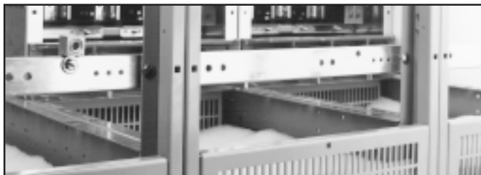
Figure 3-11 Ground Bus in Cable Compartment
