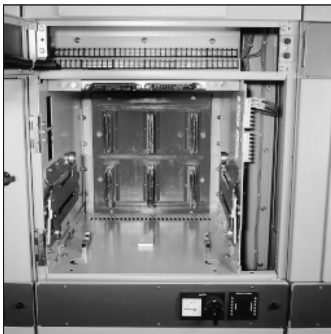
Figure 3-4 Magnum DS Breaker Cell
